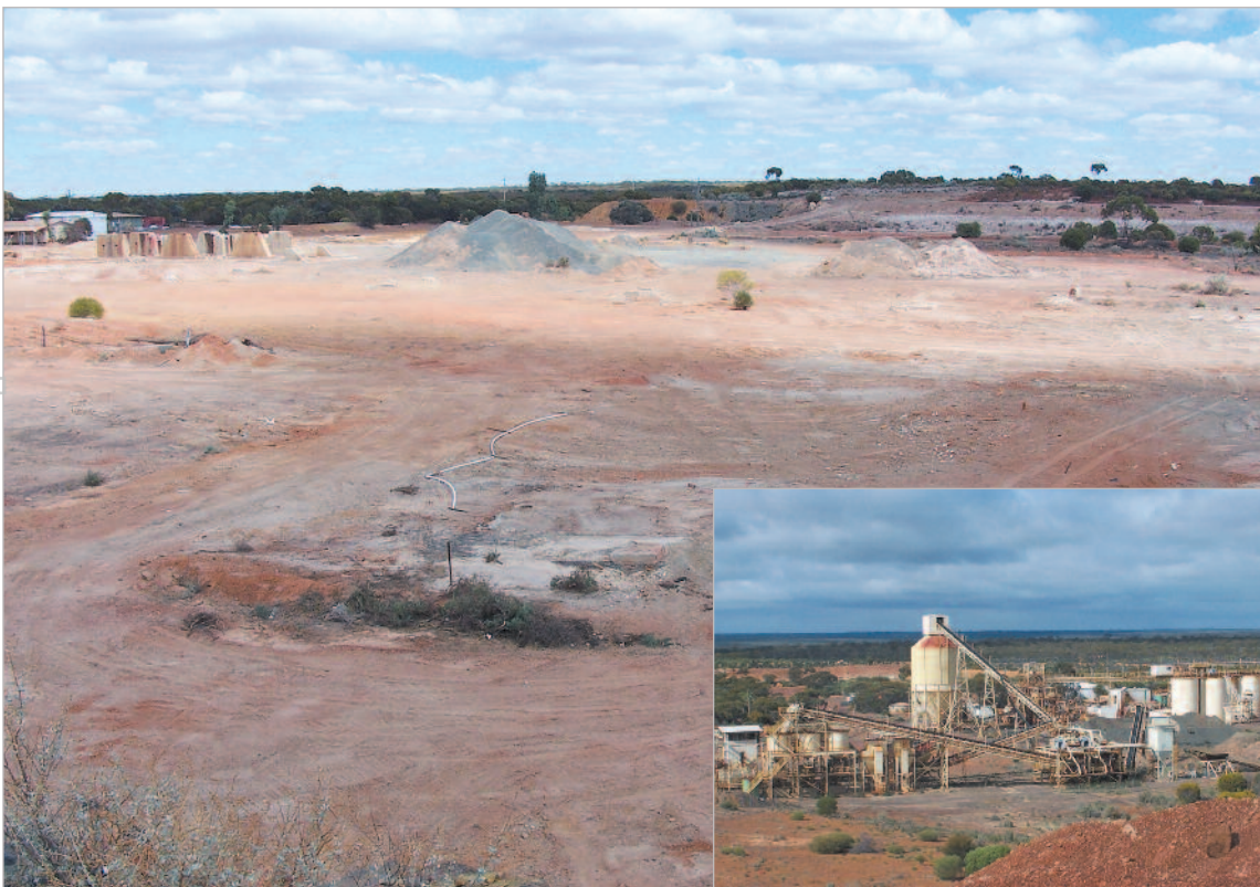
MILL SITE AT MT GIBSON POST DECOMMISSIONING (INSET: PRE DECOMMISSIONING)
