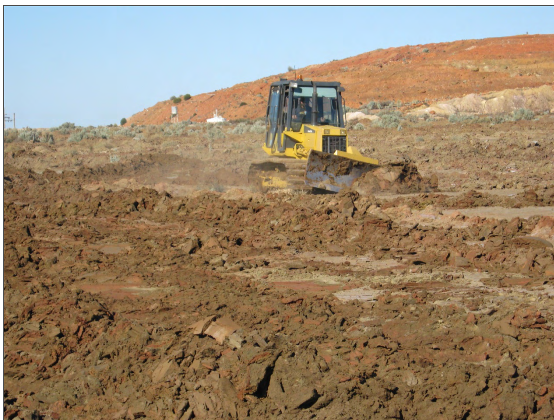
Rehabilitation activity on tailings dam – Mt Gibson
